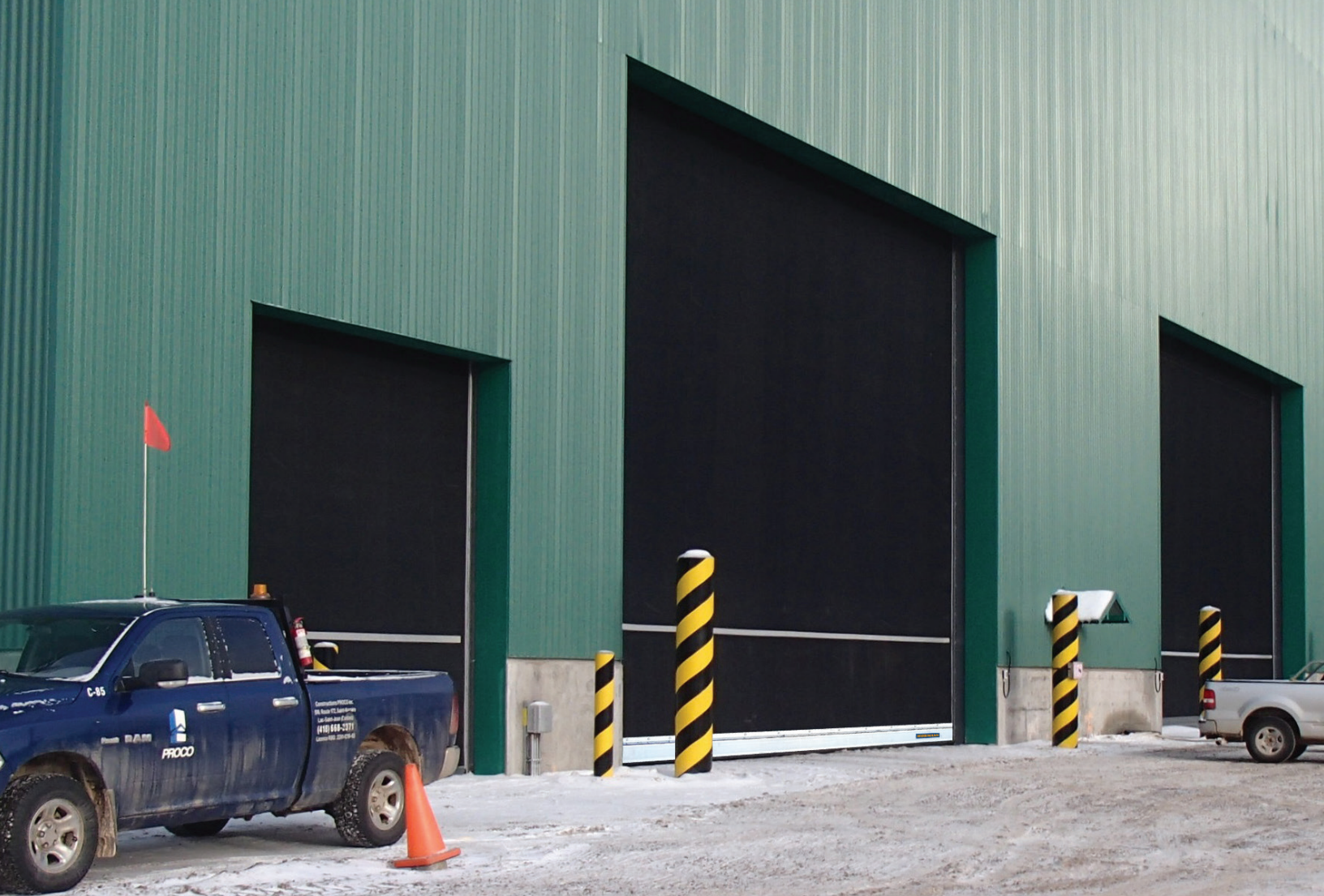
MODEL HD-CD 3025 in a mining truck maintenance shop
